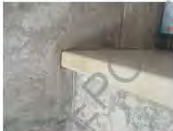
Unsealed penetration at shower seat / wall transition.
