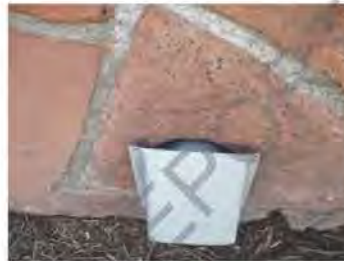
Unsealed penetration at vent.
