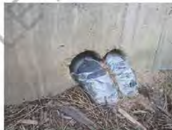
Unsealed penetration at equipment lines.
