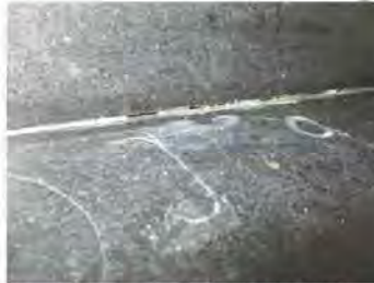
Cracked grout conditions behind sink.
