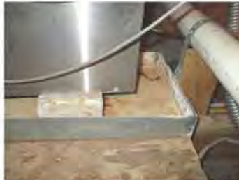
Corrosion and rust at equipment drain pan. It appears as if this overflowed at times and caused the water damage.
