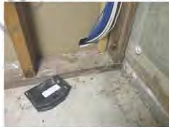
Water staining at the framing / wall.
