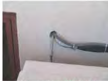
Unsealed penetration at HVAC lines.
