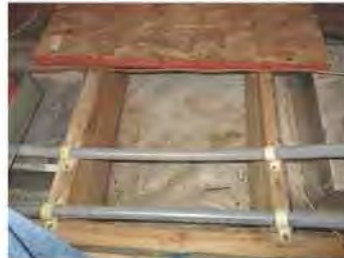
Water staining at the vapor barrier, this is believed to be the Master Shower ceiling.
