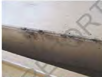
Mold-like growth at the Upper Cabinets, previously removed from the ceiling area.
