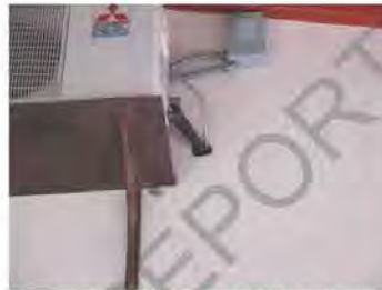
Unsealed penetration at HVAC lines.
