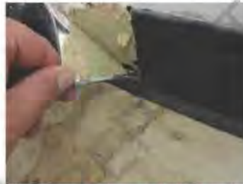
The water is tracking to the back wall, mold-like growth observed below the cove base.
