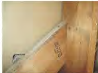
Mold-like growth at the Wall Framing.
