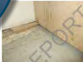
Water staining at the cabinet materials.
