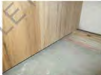
Water staining at the cabinet materials.
