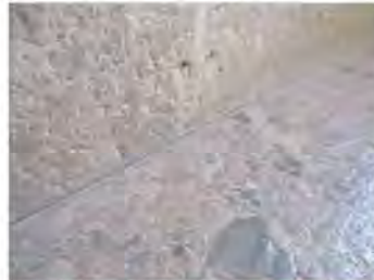
Cracked grout conditions at Tub area.
