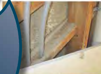
Water staining at the framing materials.
