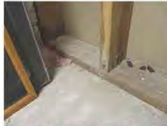
Water staining at the framing / wall.
