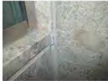
Cracked grout conditions outside of shower.
