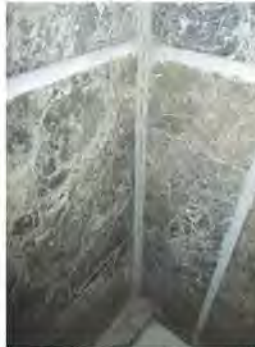
Cracked grout conditions in Shower.
