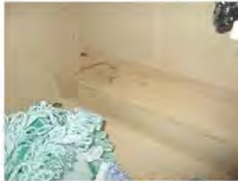
Water staining at the cabinet base below the sink.
