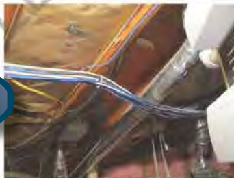
Missing insulation at roof.
