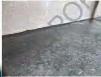
Cracked grout conditions behind sink.
