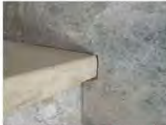
Unsealed penetration at shower seat / wall transition.
