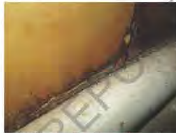
Mold-like growth at the Wall Paneling.
