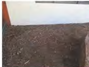
The landscaping materials are in contact with the stucco wall coverings.
