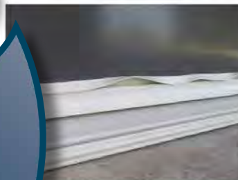
Buckled weather stripping at patio door.
