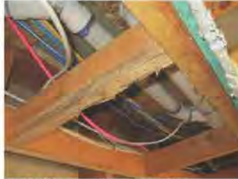
Mold-like growth at the Ceiling Framing.
