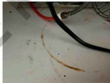
Observed some staining under the kitchen sink at the island.
