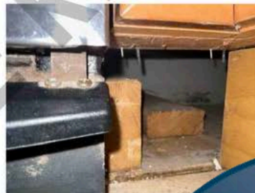
Observed mold like growth in cabinetry where the sink/dishwasher is located.
