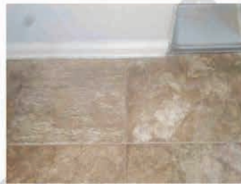
Water staining and damage observed on baseboard and flooring.
