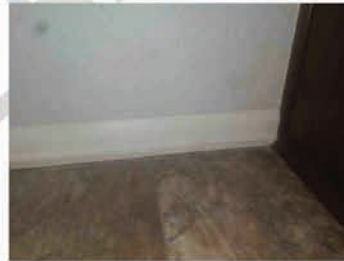
Water staining and damage observed on baseboards around shower and toilet plumbing.
